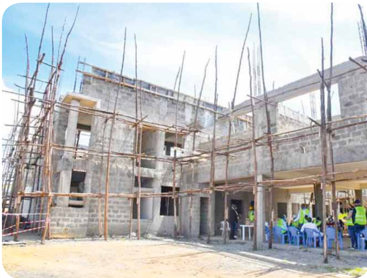
Chepterwai Hospital Complex under construction
