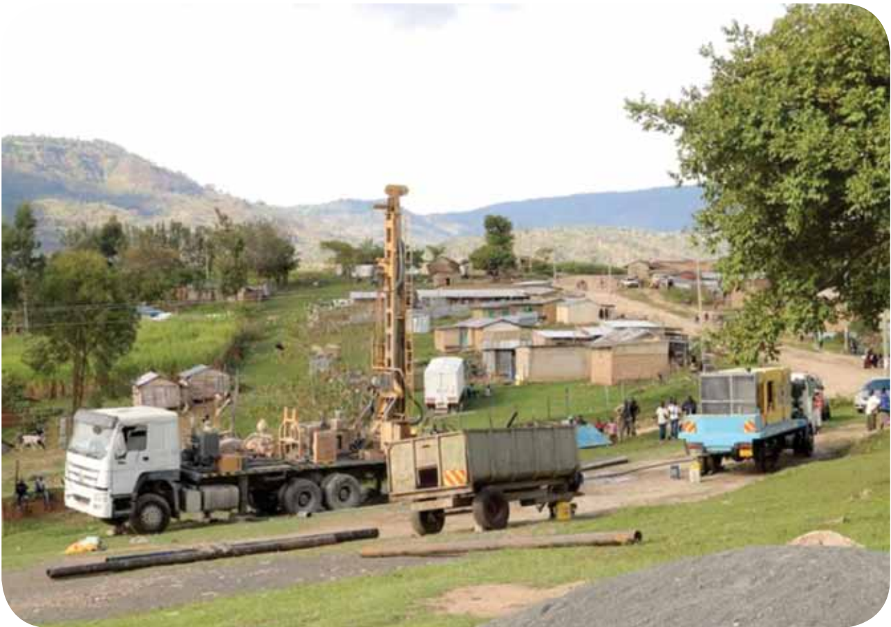
Drilling of a borehole at Tamo Primary in Sitet, Songhor-Soba ward
