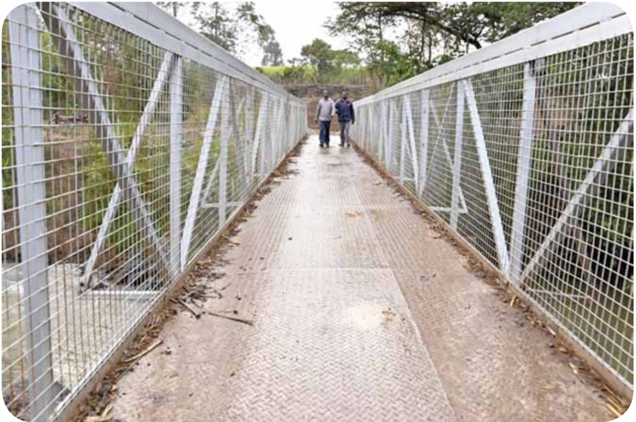
Sokyot Footbridge in Kipkaren Ward
