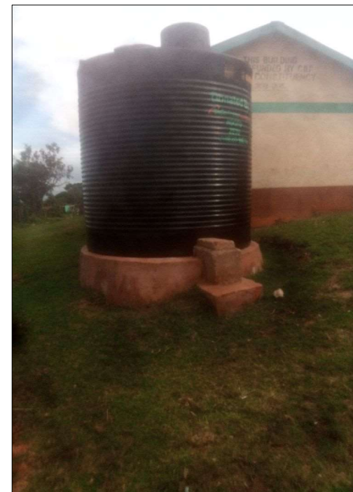
Large black tank installed with step access — used for both handwashing and drinking
