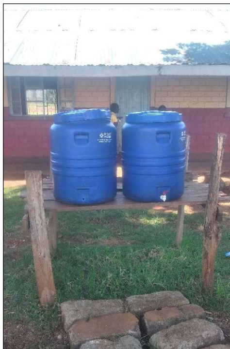
Elevated twin plastic water tanks provided by donors for improved storage capacity.
