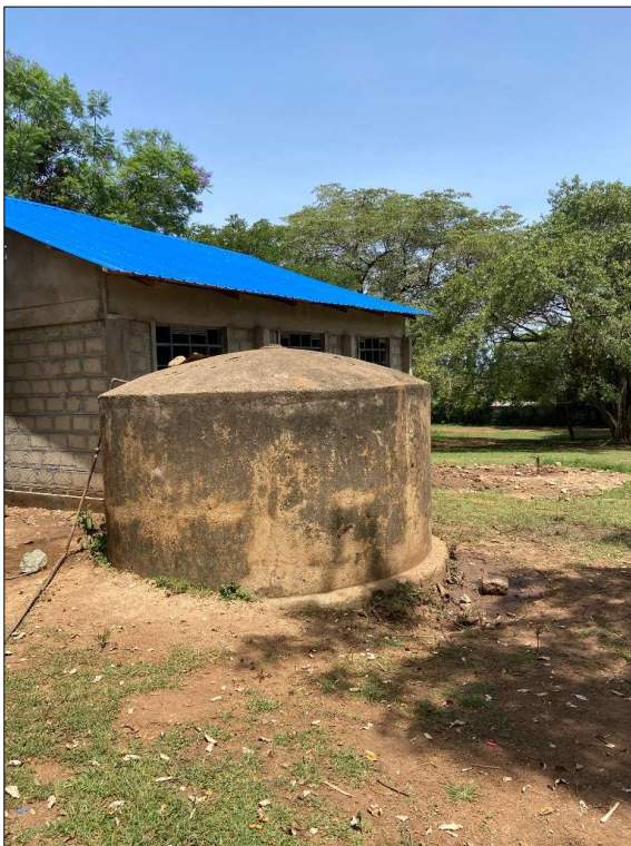
Masonry tank beside classrooms
