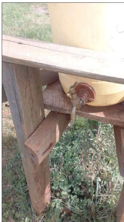
Bucket-mounted tap placed on a wooden frame — low-cost solution but limited drainage.
